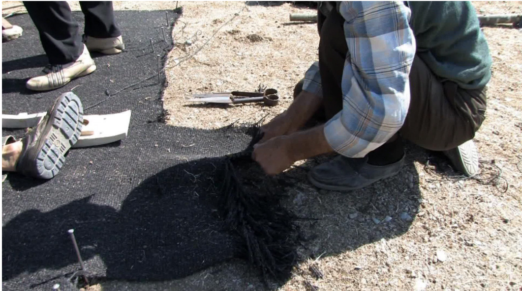
image 4.032: The flags of the centre panels can be frazzled if desired. The frazzled ends cover the ridge hole lightly, keeping off flies and allowing ventilation.
