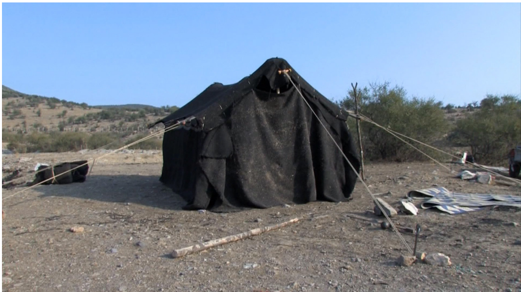
image 4.055: The finished tent. The walls were first pinned to the roof with iron nails. The surface friction of the iron was strong enough to hold the tent. Later on, wooden pins were carved out of bush twigs and replaced the metal pins. Left, in front and on the right, pieces for the second tent to be built can be seen.
