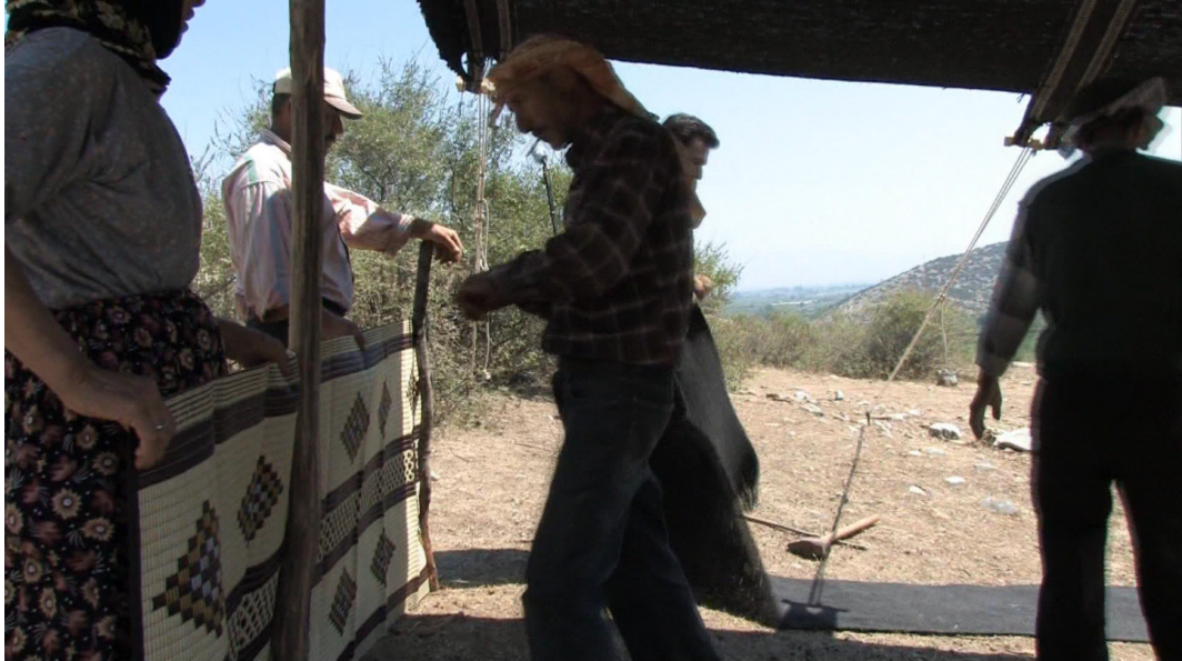
image 4.050: The wind-breaking walls are installed on the weather side of the tent. Metal bars of about 1,40 m length are driven into the ground, holding the mats upright. Each mat is sewn to the bars on two spots.
