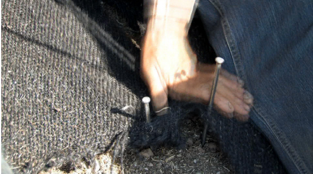
image 4.024: Abutted seam step 3. Pulling the edges together.
