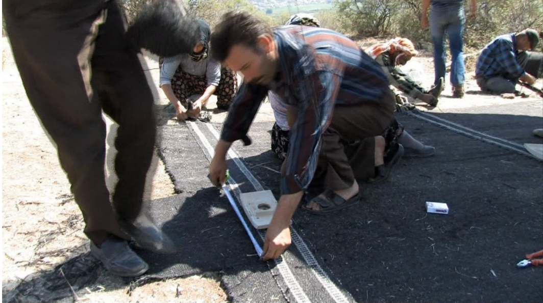
image 4.033: The ridge piece needs to be fixed exactly at the middle of the central panel.
