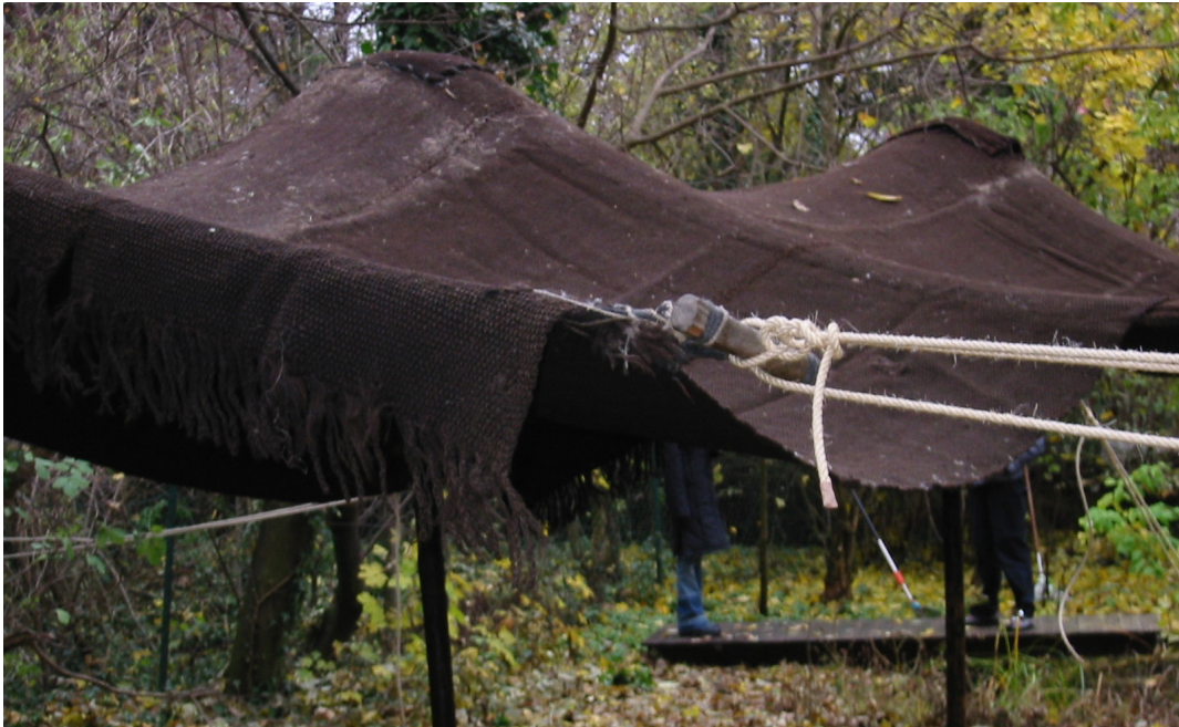
image 3.036: Final task is to fasten the guy-ropes in two steps or more by moving the 4 half-hitched knots along the leading ropes outwards. The position of the poles might need correction in some cases.
