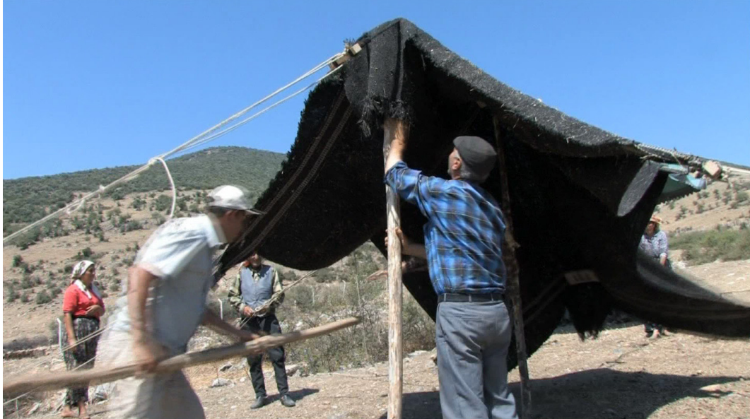
image 4.044: The whole scenery seen from the other side. The centre pole stands in place already and the last flank pole needs to be inserted. Meanwhile the front flank pole is put into an upright position. As seen, the guy-ropes are already tightly drawn, holding the unfinished tent in position. Until now, nobody had to correct the length of the guy-ropes.
