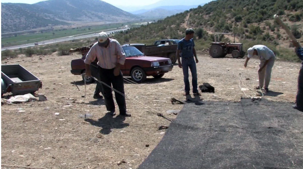
image 4.042: Just as described in chapter 3.1.4, the roof is fixed to stakes and guy-ropes before being erected.
