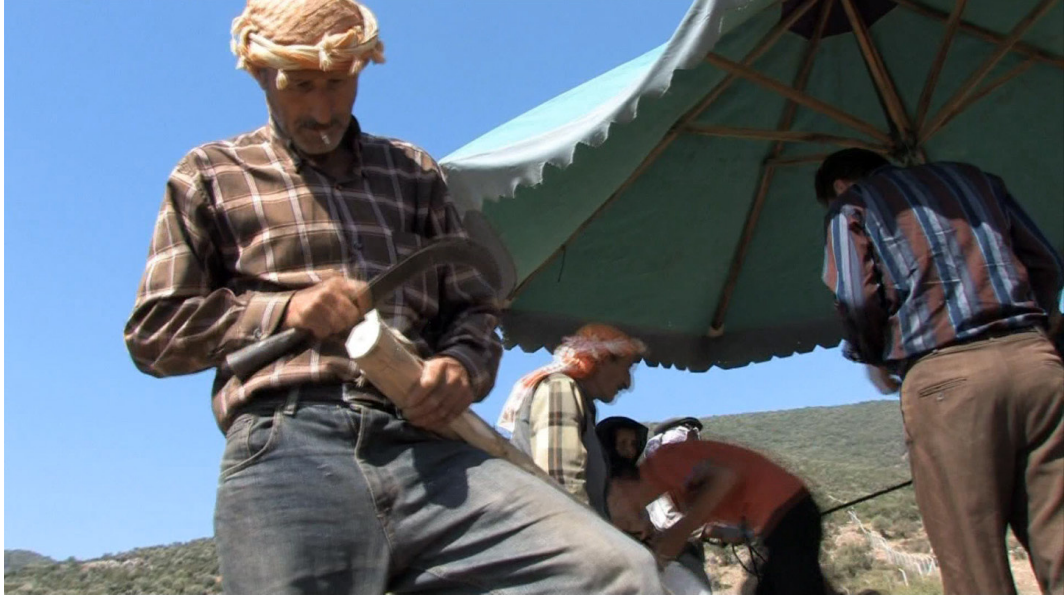
image 4.039: The heads of the poles are narrowed down with the “orak” (chop sickle) in order to fit in the trough of the ridge pieces.
