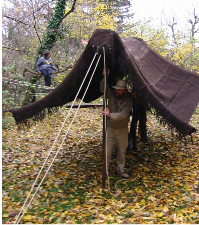
image 3.035: Further on, the poles at the flanks are set into position one by one. Again, the tent would stand on its own during the steps of erection so that a single person is able to do the whole work.
