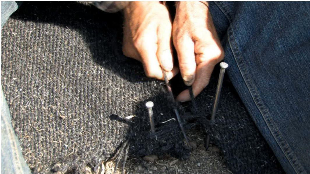
image 4.025: Abutted seam step 4. Now, the other side is stitched from underneath. All stitches must be started underneath. As seen in these pictures, “bent narrow twists” were used as needles.
