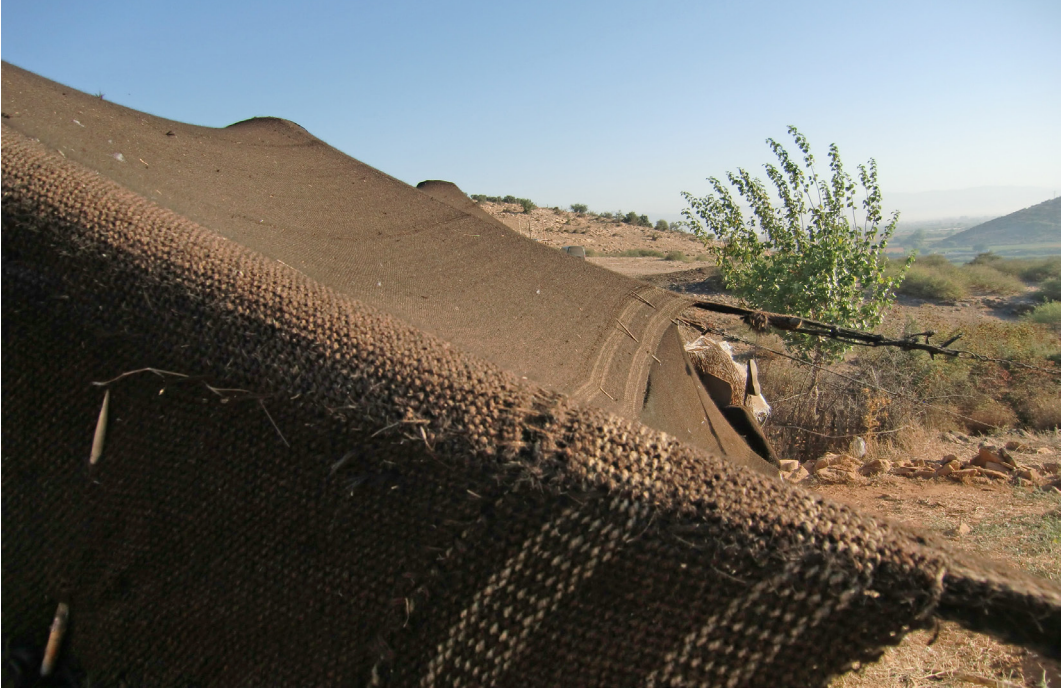
image 3.012: Yörük tent with siyek kolanı (see element “d” on the sketch after Eröz). A wooden pin (sitil çöpü or çivi) is shown left below.
