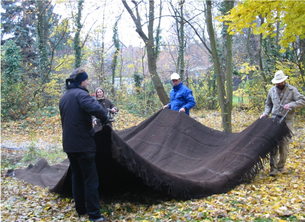
image 3.029: As already shown in the sequences for tent folding techniques, the tent roof must be spread onto the ground with the ridge pieces and ropes facing down. The position of the tent roof marks the floor plan of the to be erected tent.
