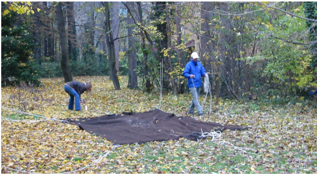
image 3.031: The guy-ropes need to be tied to the stay-fasteners being led to the stakes and back to the stay-fastener again where they get fixed with 4 half-hitched knots as shown in chapter 3.1.1. This means, that the stakes as well are driven into the ground at their estimated position before the tent is pitched up. Depending on the size of the tent, the desired wind stability and
