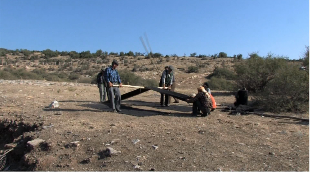
image 4.019: After the panels have been put into position, they are stretched by beating. Here, both ends of a panel are held tightly by the tent builders, while two of them raise the cloth over a horizontal pole. Another tent builder starts beating the cloth under tension with a second pole. That way, the two pole carriers and the beater slowly walk up along the panel until the whole length of it has been beaten.
