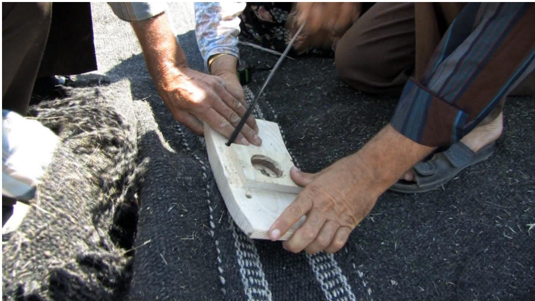
image 4.034: There, it is sewn through its 4 holes to the belt and panel. The stitch is set in a way that an "X" appears on the outside of the roof cloth. It is recommended to do the stitching several times, maybe even with separate yarns as they break easily due to friction on the wood.
