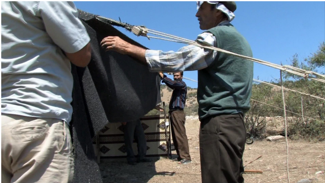
image 4.049: The length for the wall panels is measured. Afterwards, two panels for each side will be stitched together without any pre-stretching.
